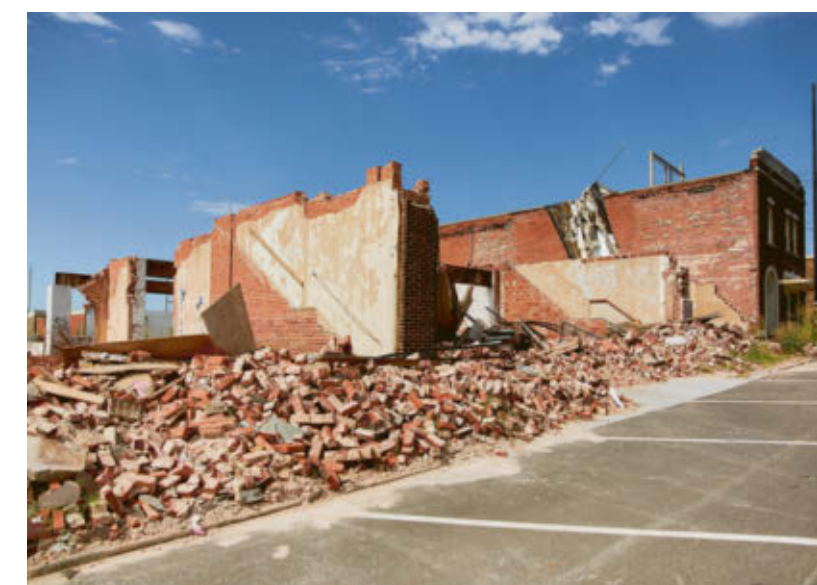
↑ Many homes in Seminole were completely destroyed by the tornados that struck the town in May.
